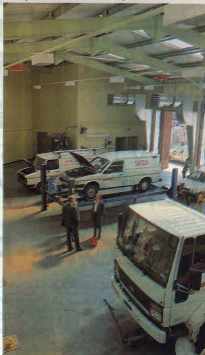
Mid-Mersey's new garage.
